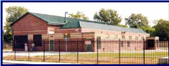
3 High Rate Treatment Facilities
