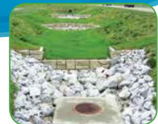
Completed Bioswale System, Florence
