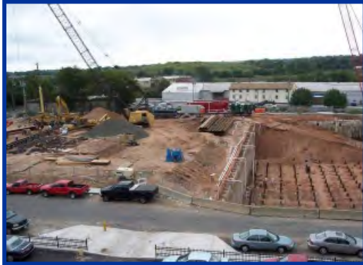
Two Underground Storage Tanks
