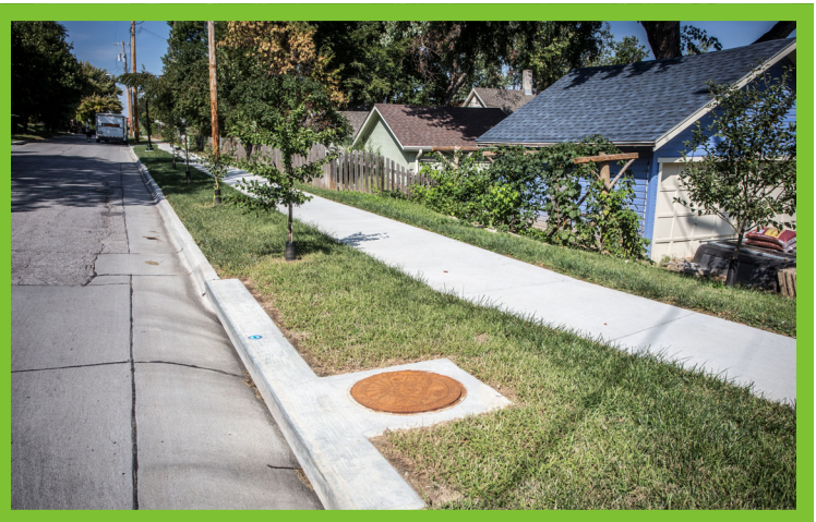
49th & Caldwell Area Sewer Separation
