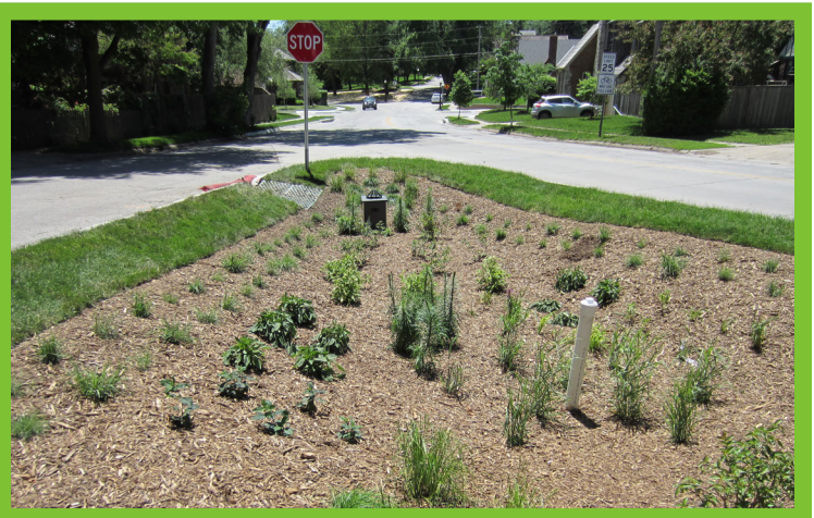
Country Club Phase 2 Sewer Separation
