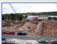
Two Underground Storage Tanks
