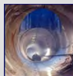
One Large Stormwater Sewer
