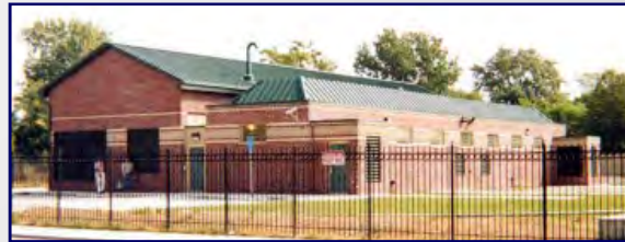
Two High-Rate Treatment Facilities
