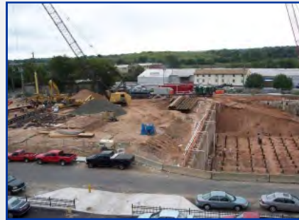
Two Underground Storage Tanks
