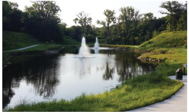
**Prior to its renovation, the park was a dumping ground for trash and yard waste. The pond now holds storm water runoff from areas where sewer separation has already been completed and has specially designed filters at inflow points.**
