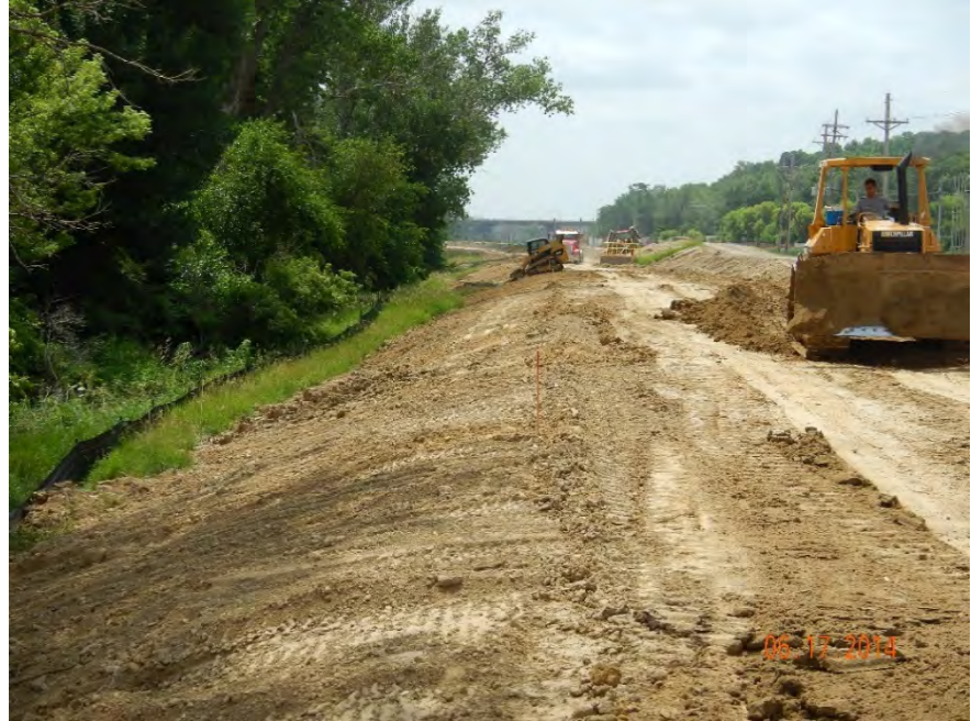
FIGURE 2-6 Construction of the SIFM South Segment (photo courtesy of HDR)
