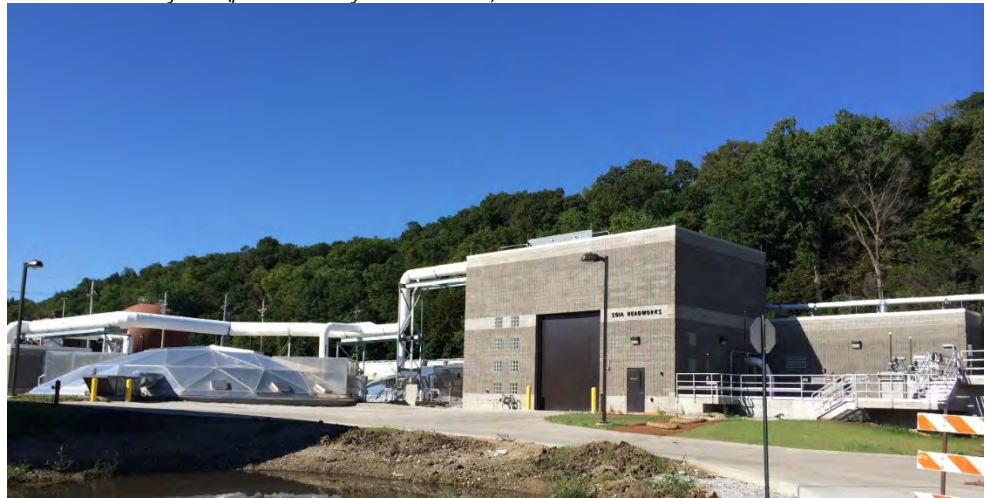
FIGURE 2-2 SOIA Treatment System (photo courtesy of CH2M HILL)
