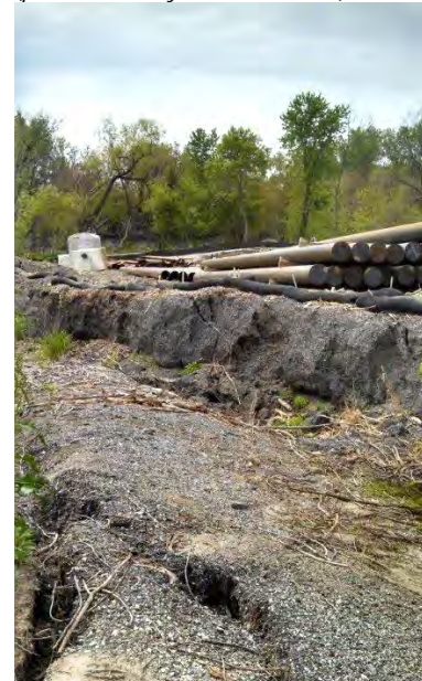
FIGURE 1-4 Unstable River Bank Conditions at the MRWWTP Site (photo courtesy of CH2M HILL)
