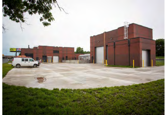
South Omaha Industrial Area Lift Station (photo courtesy of Wade Trim)
