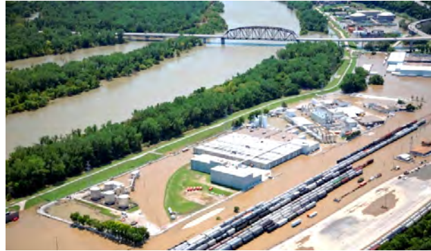
FIGURE 1-3 Flooding in 2011 near the MRWWTP (photo courtesy of City of Omaha)
