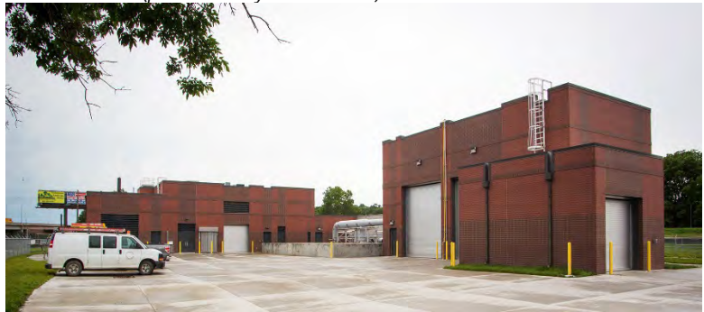
FIGURE 2-1 SOIA Lift Station (photo courtesy of Wade Trim)
