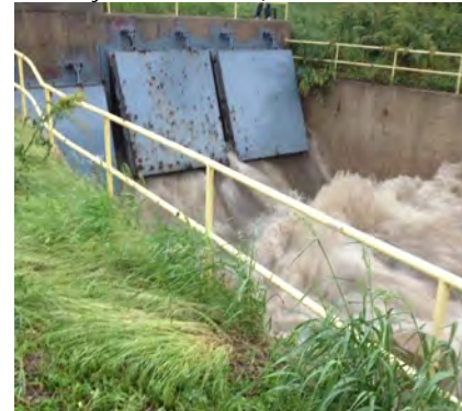
FIGURE 3-9 Discharge from CSO 105 during the June 3, 2014 Storm Event (photo courtesy of CH2M HILL)
