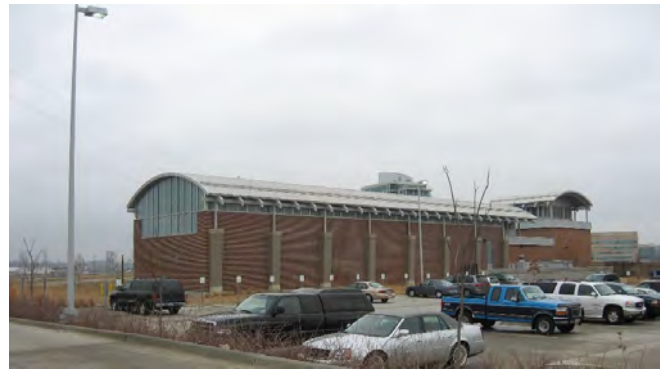
FIGURE 3-4 Burt Izard Lift Station
