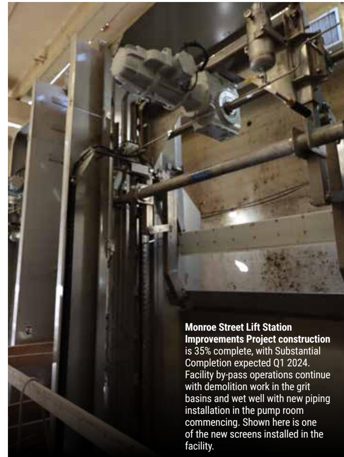
**Monroe Street Lift Station Improvements Project** construction is 35% complete, with Substantial Completion expected Q1 2024. Facility by-pass operations continue with demolition work in the grit basins and wet well with new piping installation in the pump room commencing. Shown here is one of the new screens installed in the facility.
