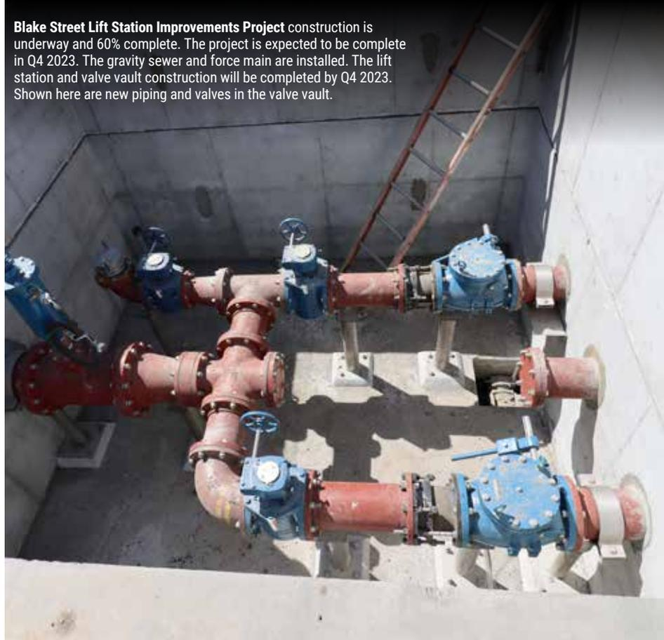
**Blake Street Lift Station Improvements Project** construction is underway and 60% complete. The project is expected to be complete in Q4 2023. The gravity sewer and force main are installed. The lift station and valve vault construction will be completed by Q4 2023. Shown here are new piping and valves in the valve vault.
