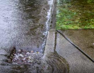
During heavy rain or snow events, stream and stormwater runoff rushes into nearby gutters and storm drains that lead to the sewer system. If the system reaches or exceeds capacity, basement backups or street flooding can occur, causing hazardous conditions.
